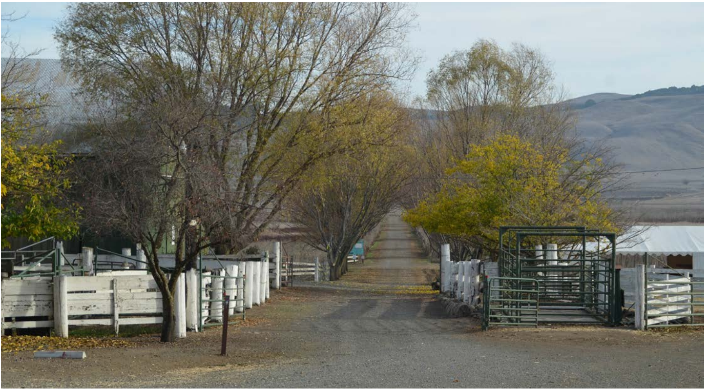
East-Facing View of the Tolay Lake Causeway
