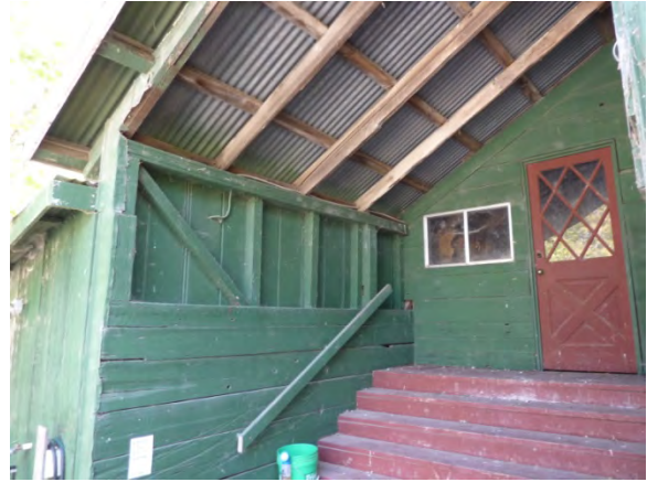
Image 81 - Recessed entrance at north elevation
