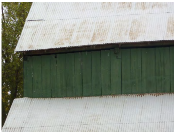
Image 49 - Typical condition of roof
