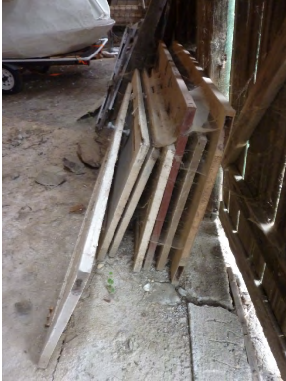
Image 120 - Cracked foundation at south wall
