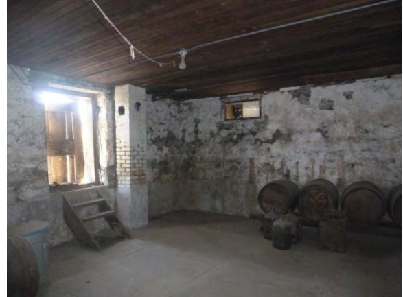
Image 68 - Interior of upper section, with wood ceiling and stone walls
