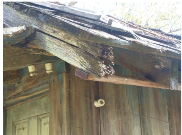
Image 98 - Roofing and structure at west side
