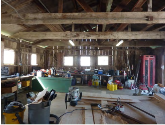
Image 124 - Interior currently being used as a workshop
