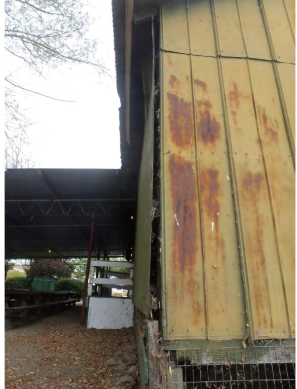
Image 89 - Typical condition of metal siding.
