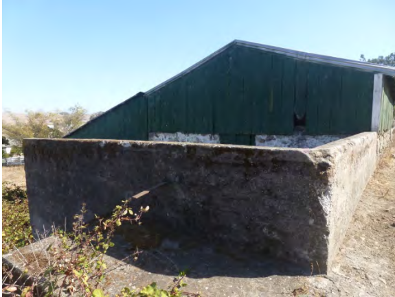
Image 67 - Concrete walls on north side of creamery
