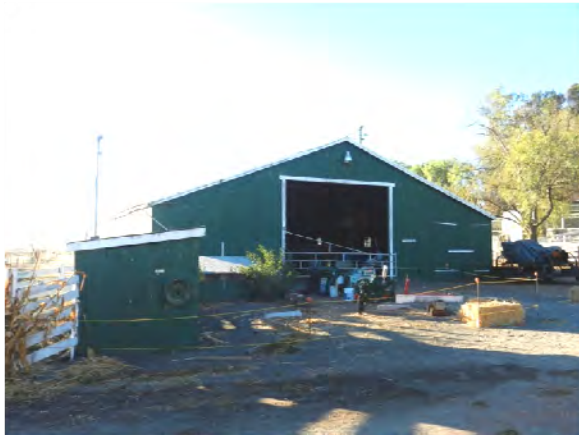
Image 113 – North entrance to Tractor Barn.
