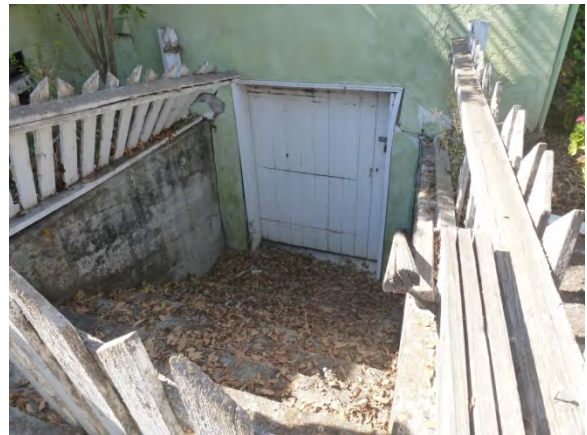
Image 21 - Stairs to basement
