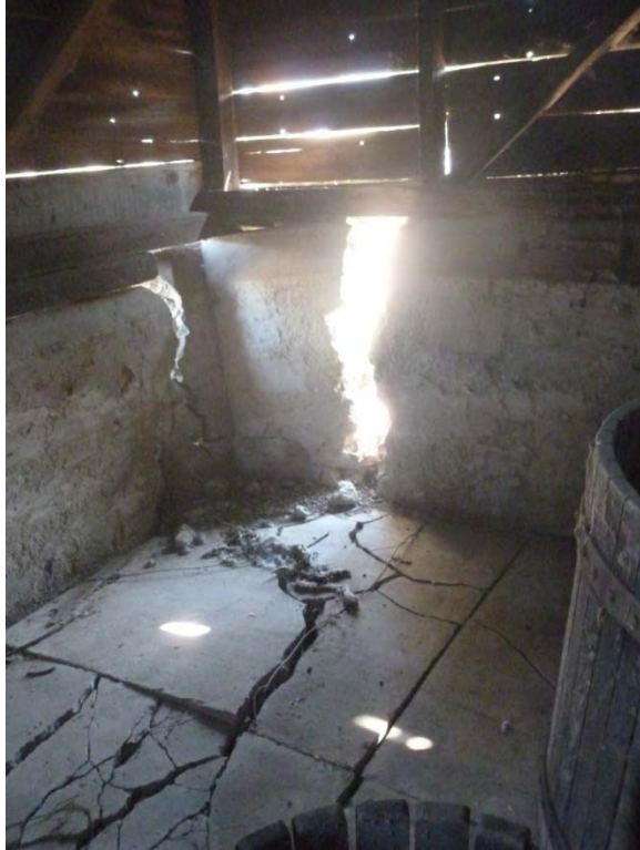
Image 77 - Condition at northeast corner.
