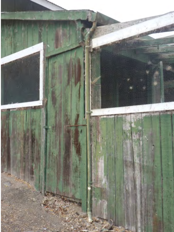
Image 88 - Typical condition of wood siding and doors to chicken coop.
