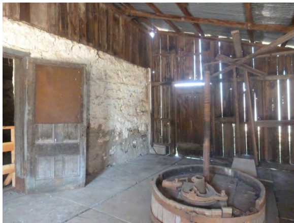
Image 75 - General condition of interior
