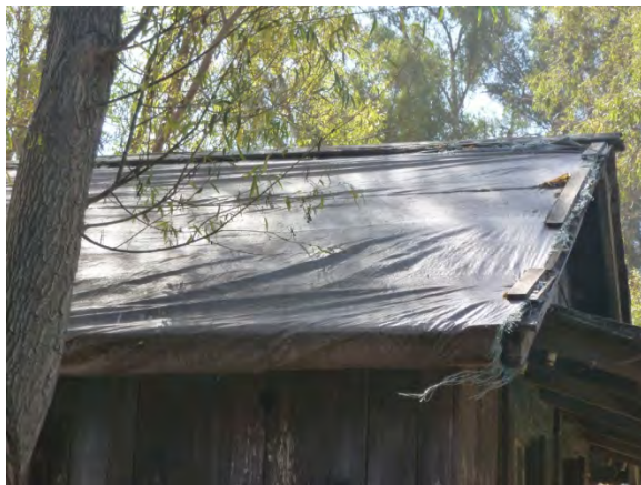
Image 97 - Tarp-clad east side of roof
