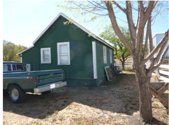
Image 2 – Northeast corner of Cottage
