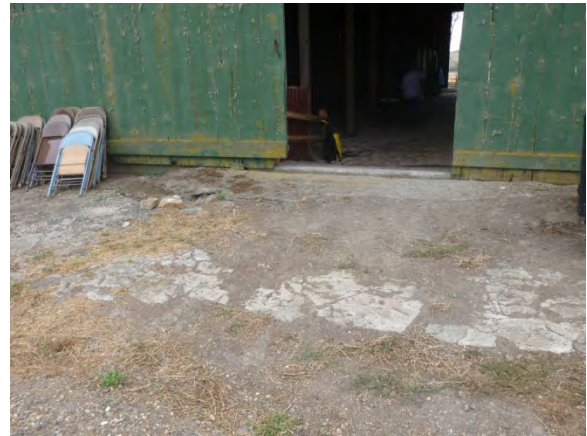
Image 54 – Stone and concrete paving at north entrance
