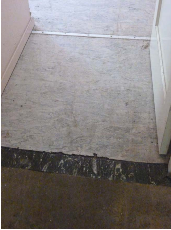
Image 22 - Multiple layers of flooring
