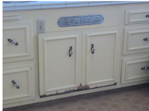
Image 43 - Cabinet at kitchen sink
