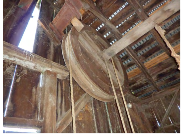
Image 135 - Winch and tackle near southeast corner
