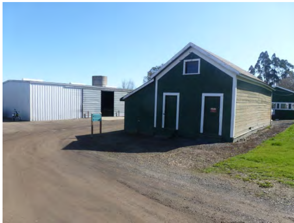
Image 102 – North wall of Old Shop
