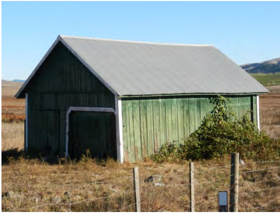
Image 132 – Entrance in west wall of Slaughterhouse
