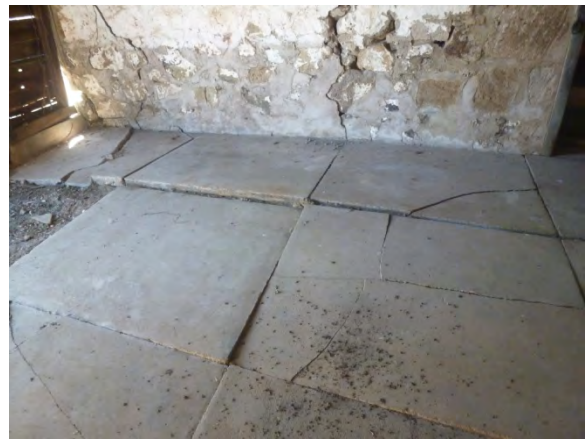
Image 76 - Floor slabs at mid-level of building
