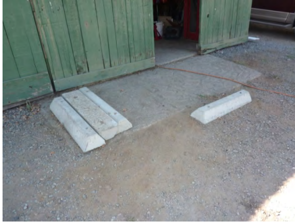
Image 126 – Entrance to working space in Storage Shed
