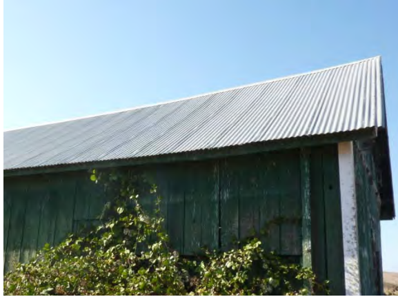
Image 136 - General condition of roofing.
