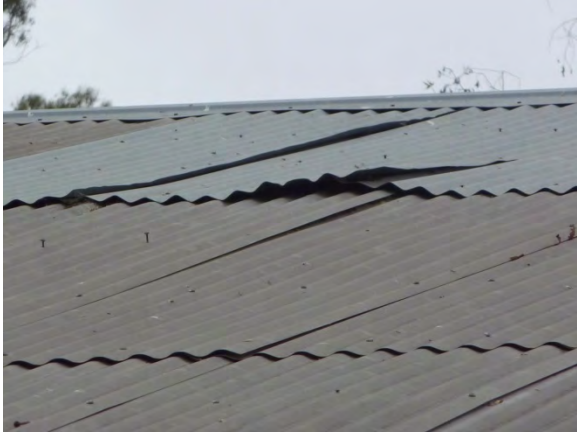
Image 116 - Typical condition of roofing
