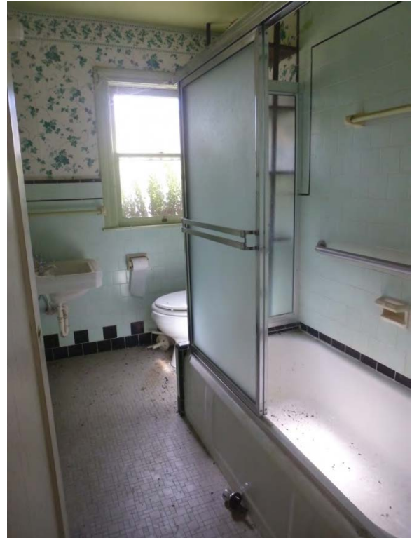
Image 14 - Bathroom with original tile and fixtures
