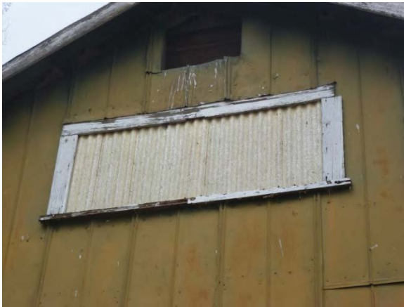
Image 90 - South Gable window with fiberglass infill.
