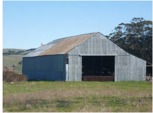
Image 58 – West entrance to Old Dairy Barn
