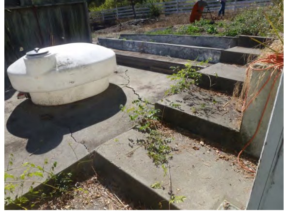
Image 16 - Terraced patio on south side of garage
