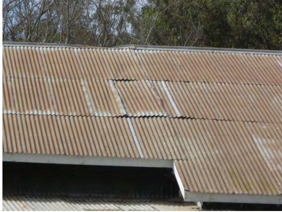
Image 86 - General condition of roofing
