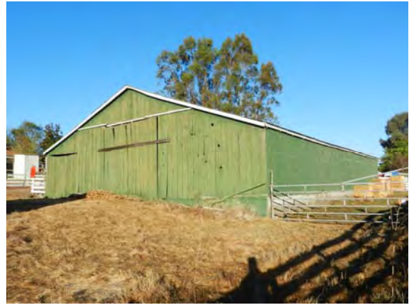
Image 114 – Southeast corner of Tractor Barn.
