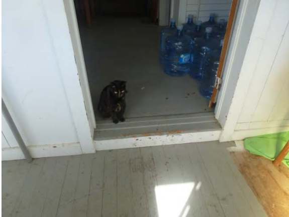
Image 8 - Step between enclosed porch and cottage
