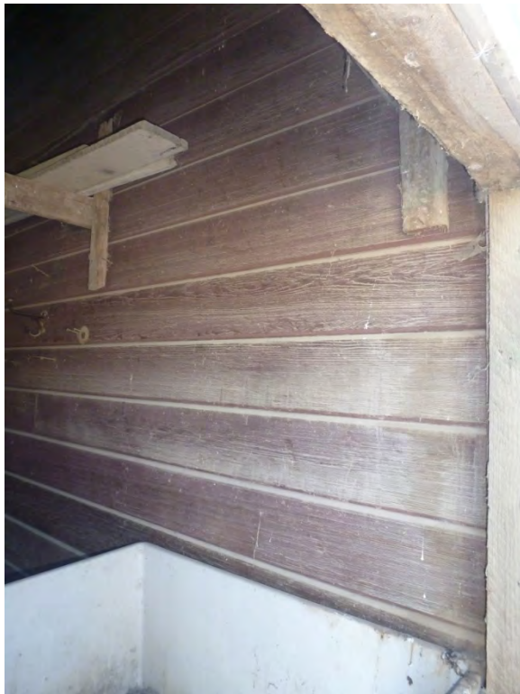
Image 106 - Original exterior wall within shed
