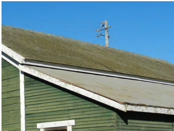
Image 108 - Typical condition of roofing
