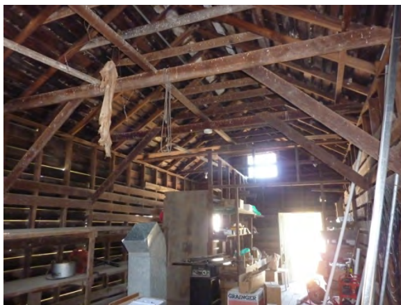
Image 104 - Interior of workshop
