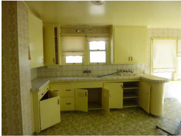
Image 12 - Kitchen with original cabinets and counters
