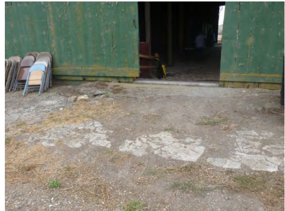
Image 54 – Stone and concrete paving at north entrance
