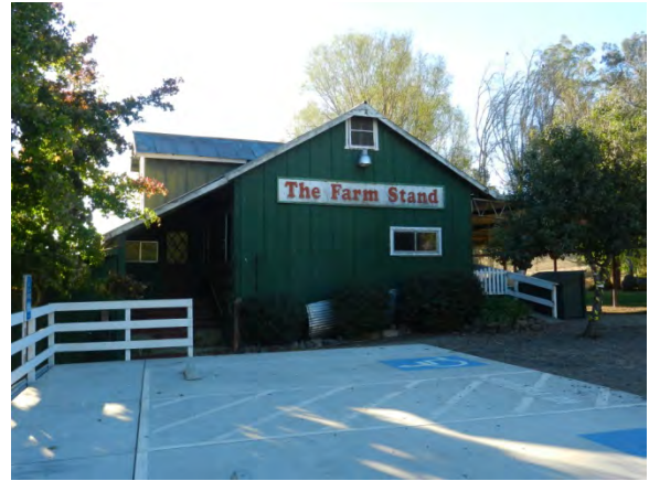
Image 79 – North end of Granary
