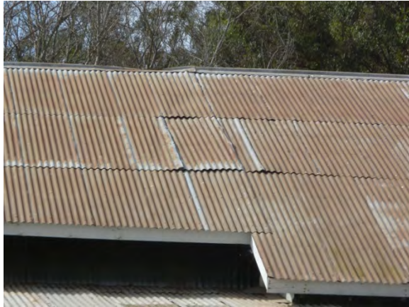
Image 86 - General condition of roofing
