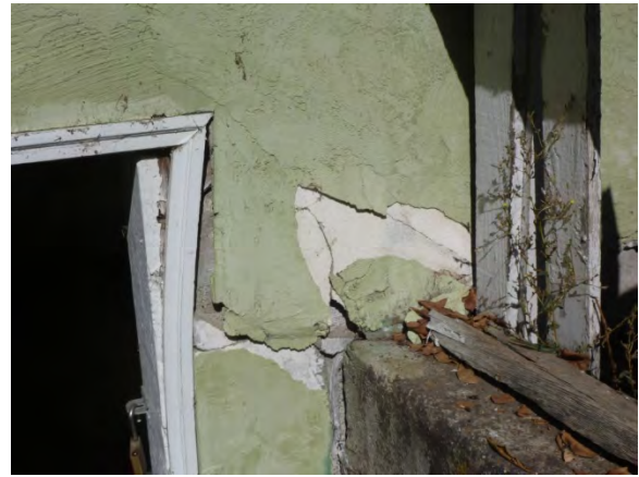
Image 18 - Stucco at basement stair and door
