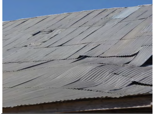
Image 63 - Sheet Metal Roofing
