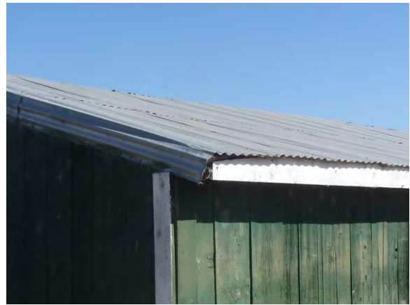
Image 71 - Metal Roofing, wrapped at gable end
