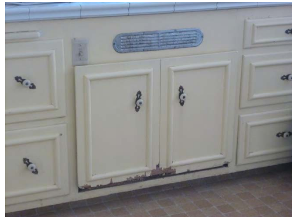
Image 43 - Cabinet at kitchen sink
