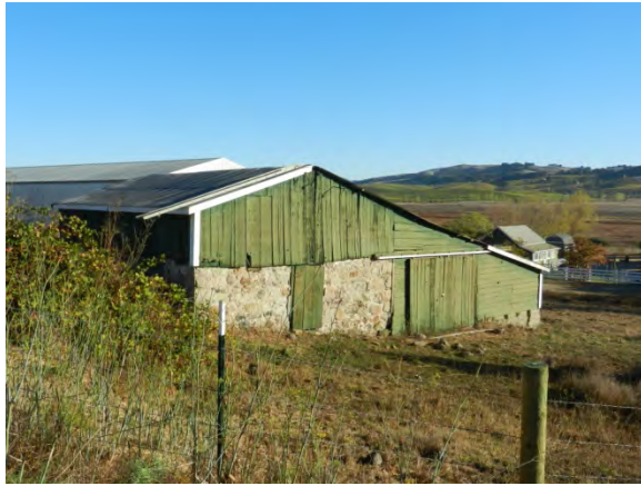
Image 65 – South wall of Creamery
