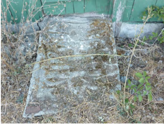
Image 134 - Concrete drainage trough at east end of building
