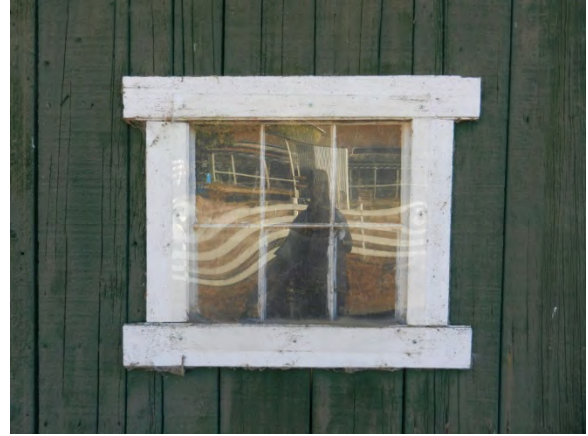
Image 119 - Typical window with plexiglas cover
