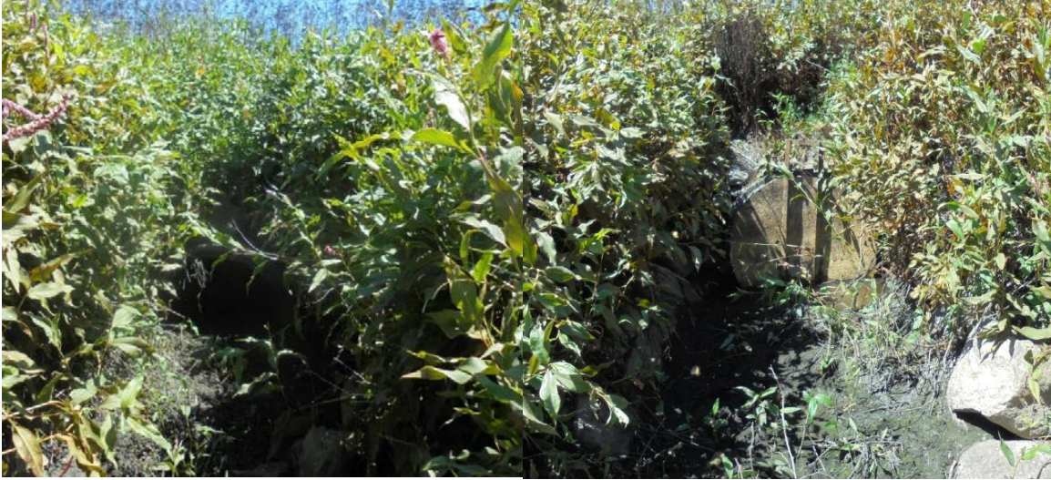
Figure 4. Closed gated culvert in horseshoe berm, inlet shown on left, outlet shown on right.
