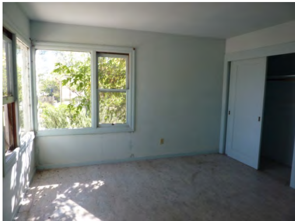
Image 13 - Bedroom in addition
