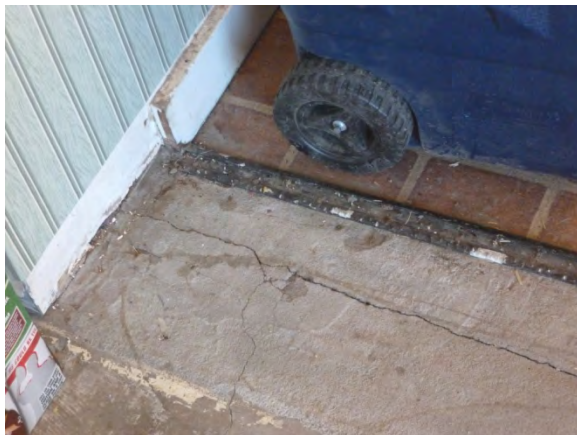
Image 41 - Floor at former garage
