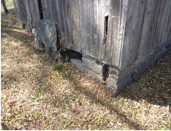
Image 99 - Building set on wood skids directly on ground
