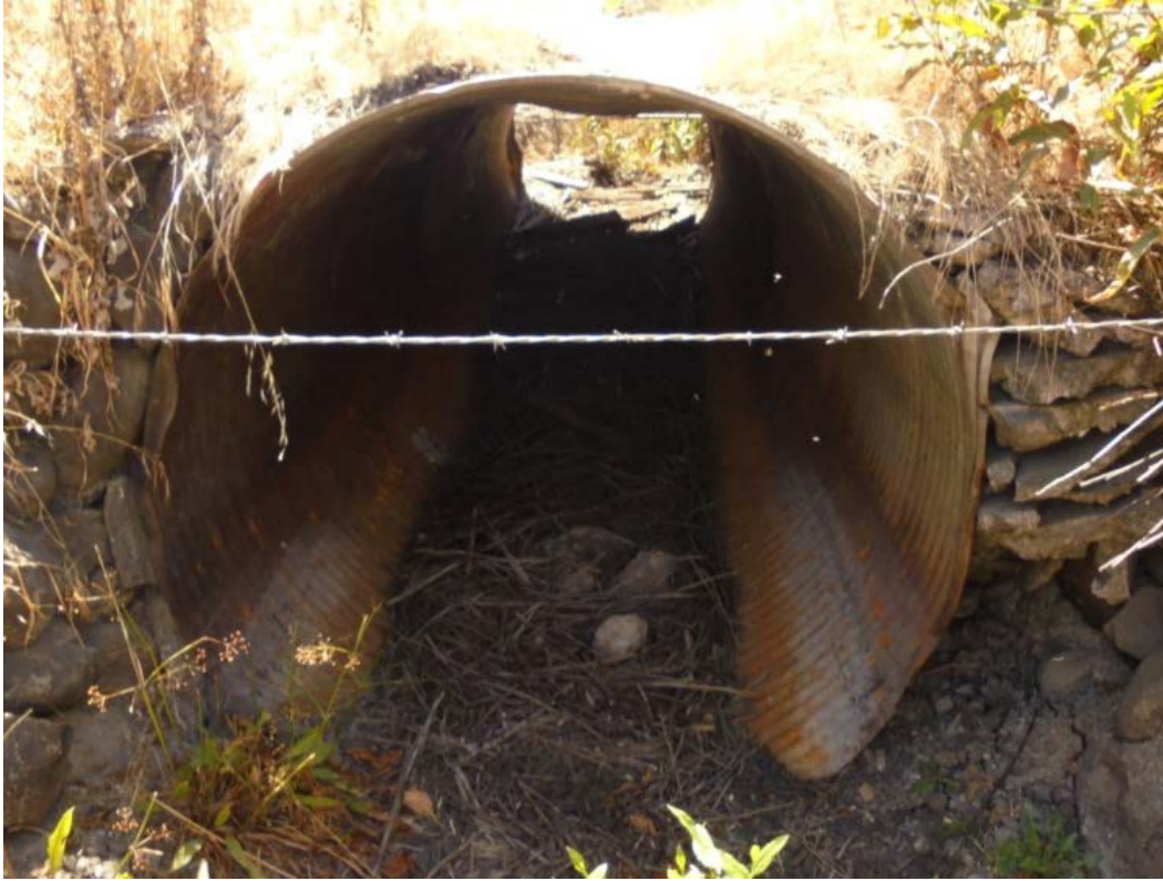
Figure 6. East Channel Causeway Culvert inlet.
