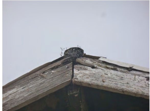
Image 87 - Roofing and trim at ridge, south end
