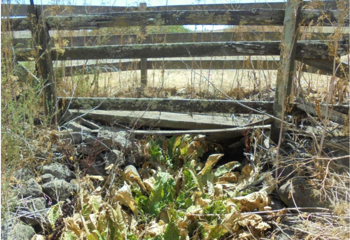
Figure 2. West Channel Causeway Culvert inlet.
