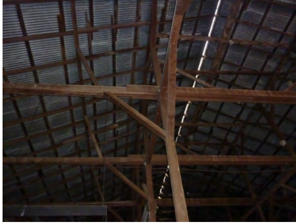
Image 47 - Barn framing and open vent at ridge
