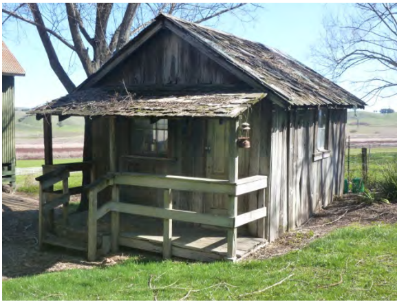
Image 96 – Front of Line Shack, facing north, leaning toward west
