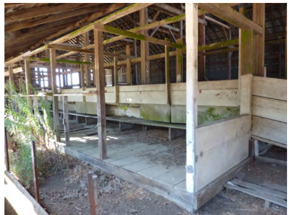
Image 64 - Stalls inside barn
