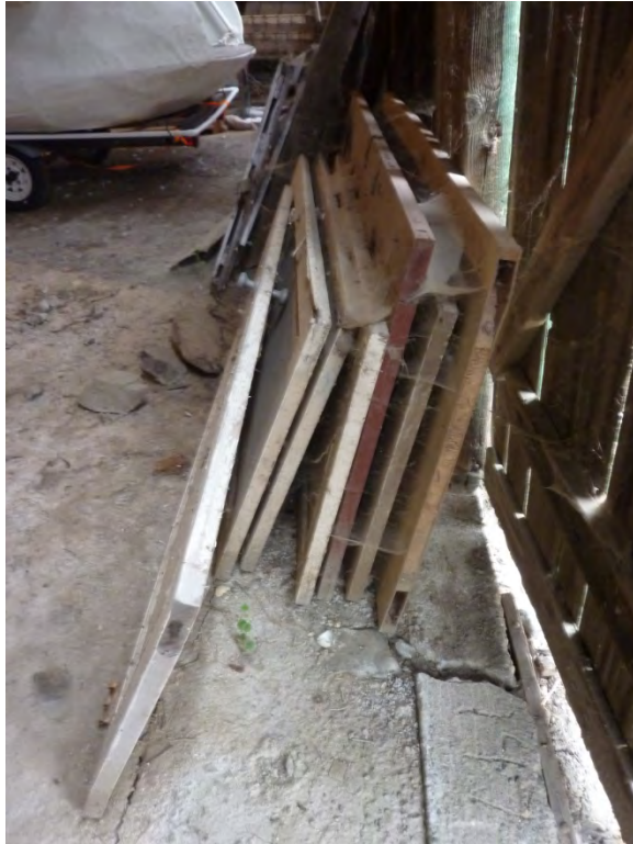
Image 120 - Cracked foundation at south wall
