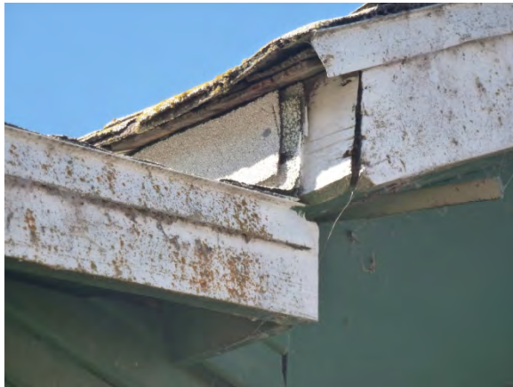
Image 5 - Enclosed porch roof at Cottage
