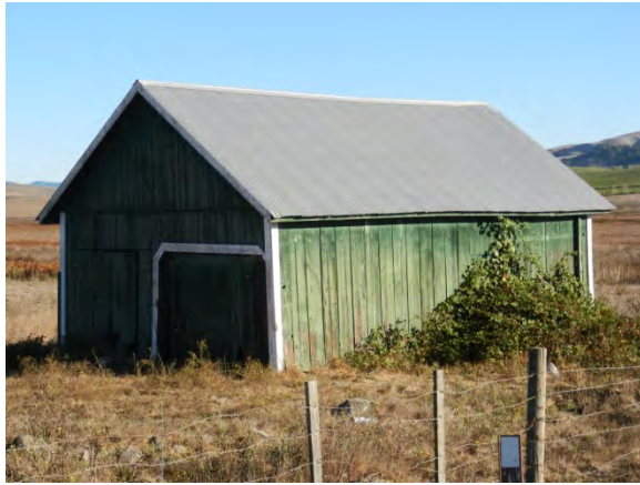
Image 132 – Entrance in west wall of Slaughterhouse
