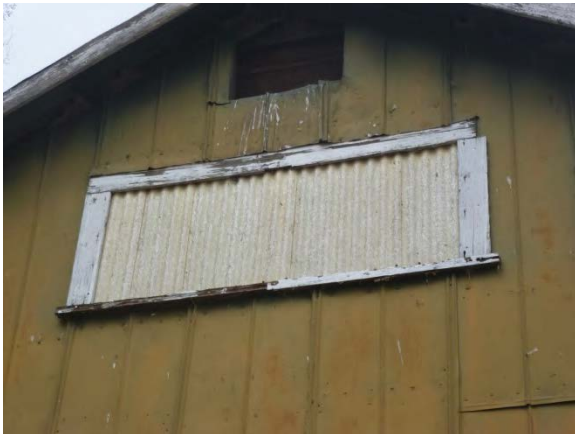
Image 90 - South Gable window with fiberglass infill.
