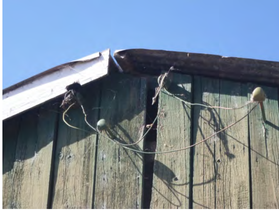
Image 72 - Condition at ridge
