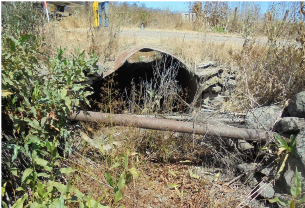
Figure 7. East Channel Causeway Culvert outlet.
