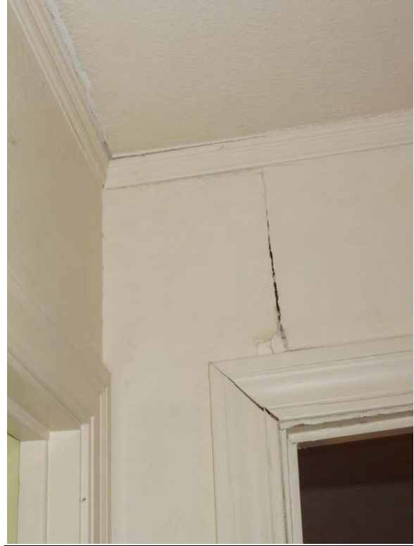
Image 23 - Settlement damage
