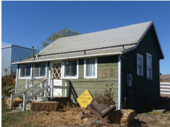
Image 1 - Entrance to Cottage, south side
