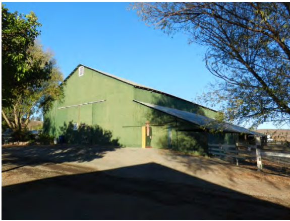
Image 45 – South wall of Hay Barn with shed on right
