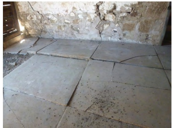
Image 76 - Floor slabs at mid-level of building
