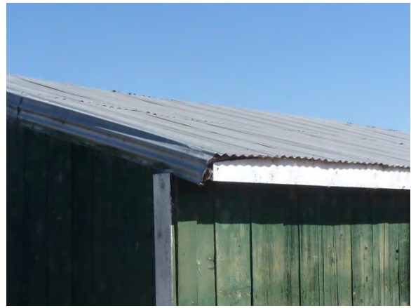
Image 71 - Metal Roofing, wrapped at gable end
