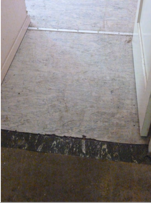
Image 22 - Multiple layers of flooring
