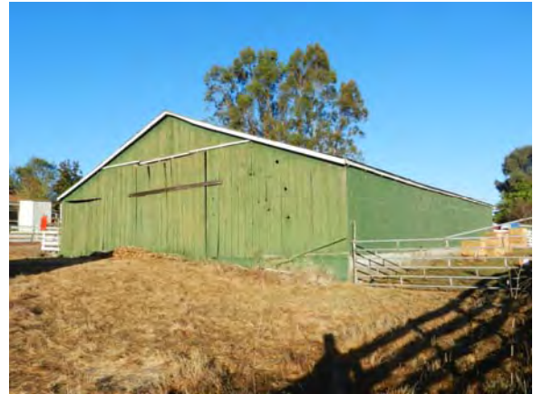
Image 114 – Southeast corner of Tractor Barn.
