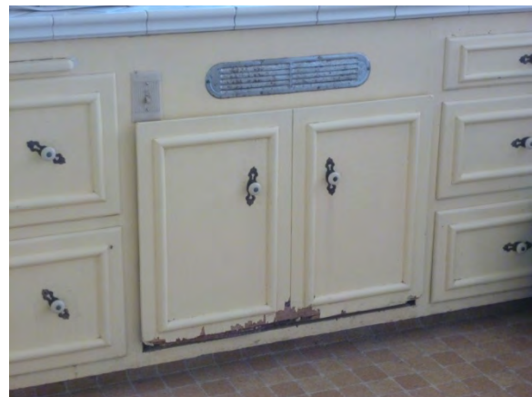
Image 43 - Cabinet at kitchen sink
