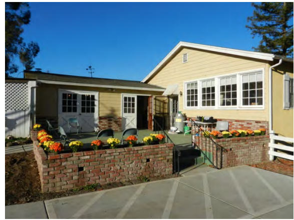
Image 28 - John Jr. and Beatrice’s House, with addition and garage at south end
