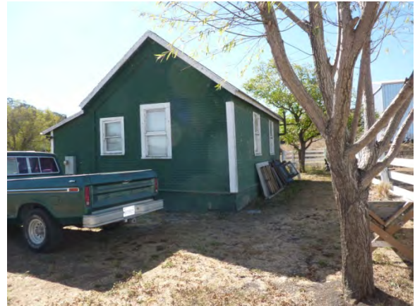
Image 2 – Northeast corner of Cottage
