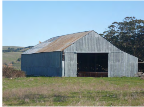
Image 58 – West entrance to Old Dairy Barn
