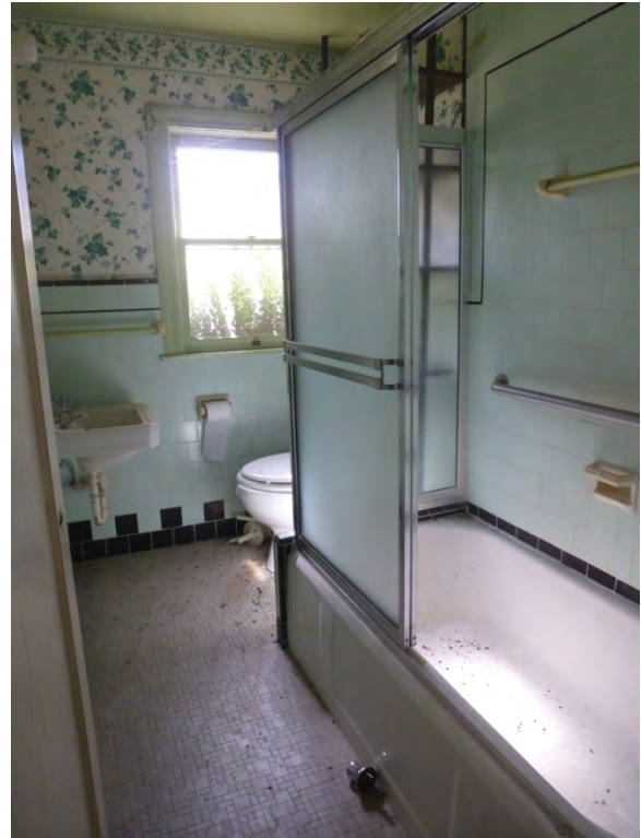
Image 14 - Bathroom with original tile and fixtures
