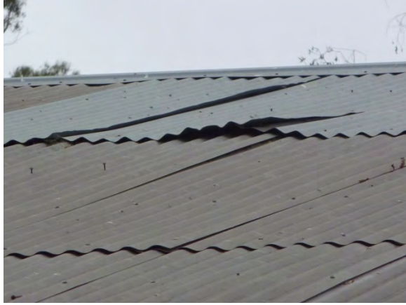
Image 116 - Typical condition of roofing
