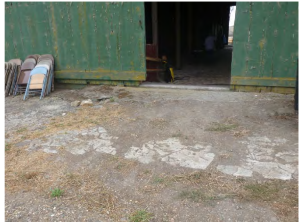
Image 54 – Stone and concrete paving at north entrance
