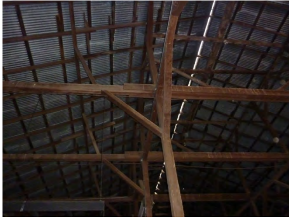
Image 47 - Barn framing and open vent at ridge
