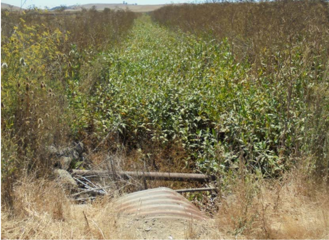
Figure 8. East Channel downstream of Causeway.
