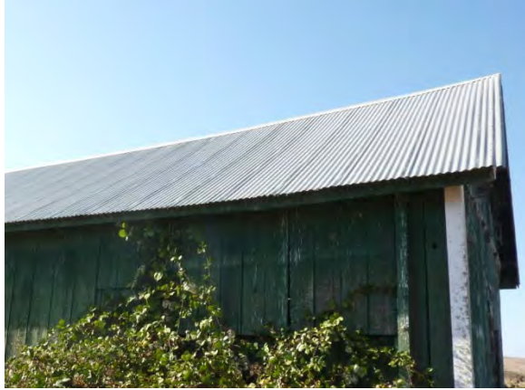
Image 136 - General condition of roofing.
