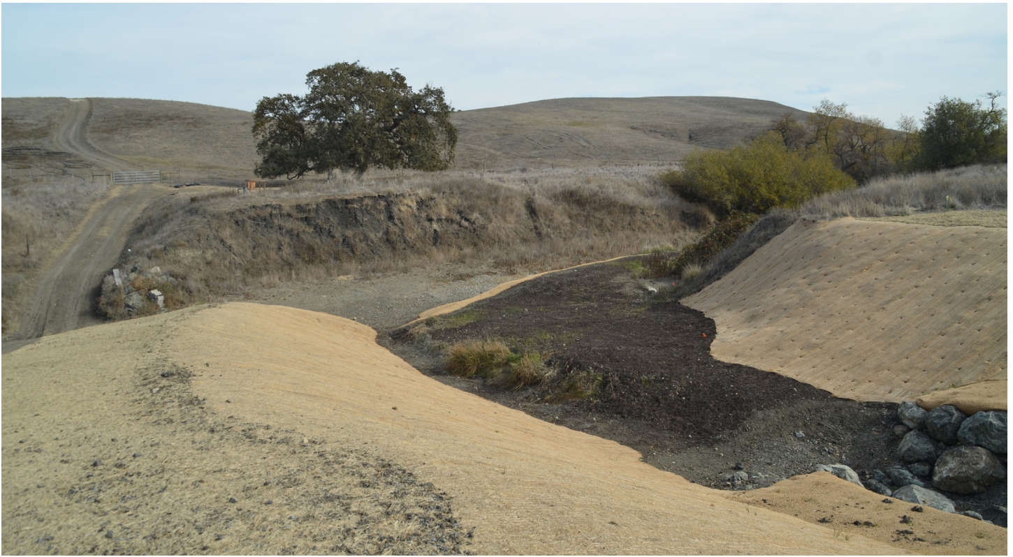
South Entrance Staging Area (Background)
