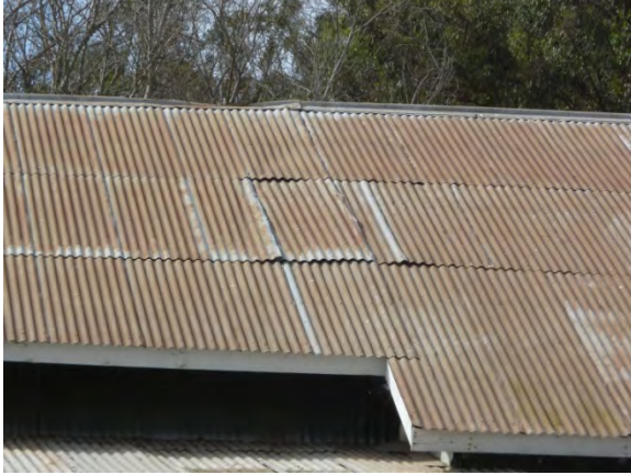
Image 86 - General condition of roofing
