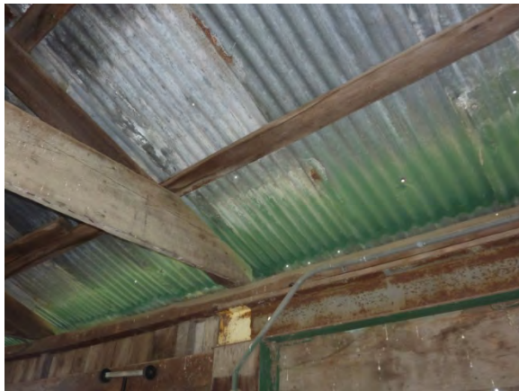
Image 129 - Corrugated roofing and steel beam at door
