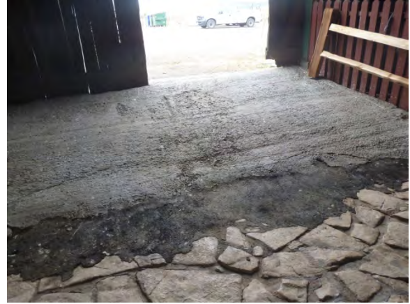
Image 56 - Stone floor with concrete topping at south entrance
