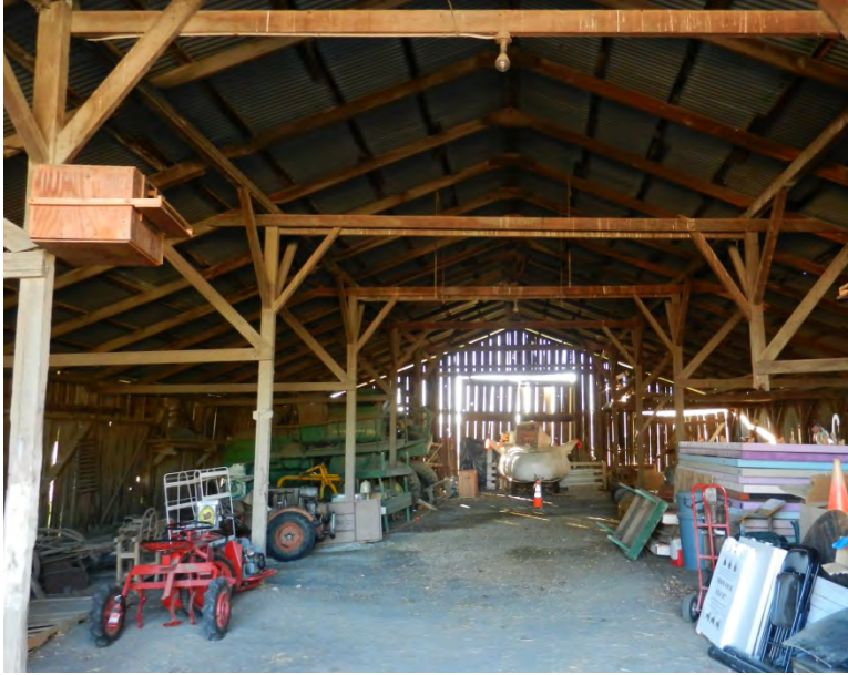
Image 115 - Barn interior showing framing and dirt floor
