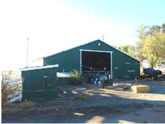
Image 113 – North entrance to Tractor Barn.
