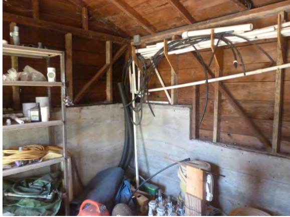
Image 15 - Interior of garage showing stepped foundation walls
