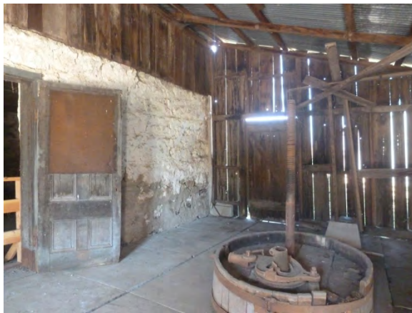
Image 75 - General condition of interior
