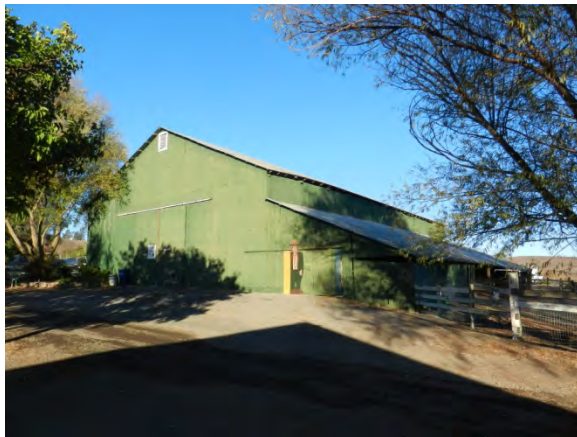
Image 45 – South wall of Hay Barn with shed on right
