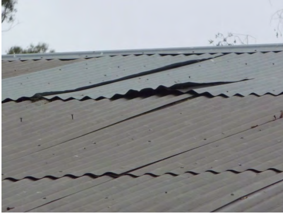
Image 116 - Typical condition of roofing
