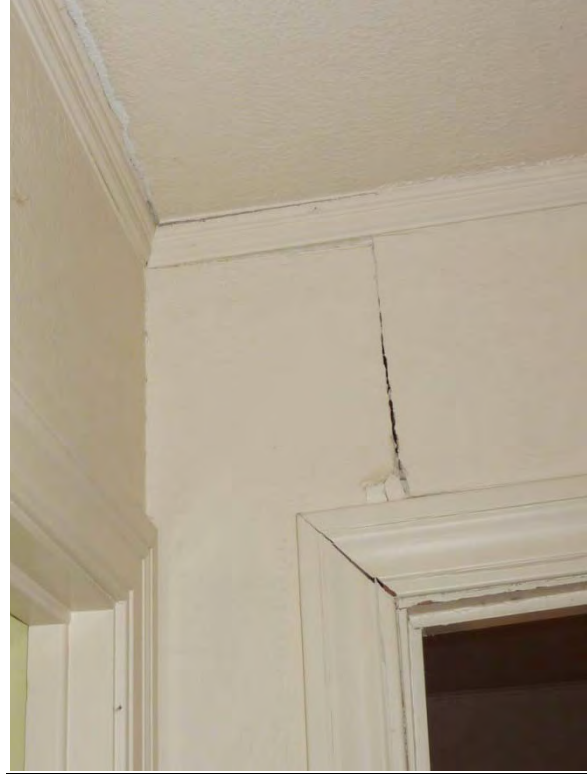
Image 23 - Settlement damage
