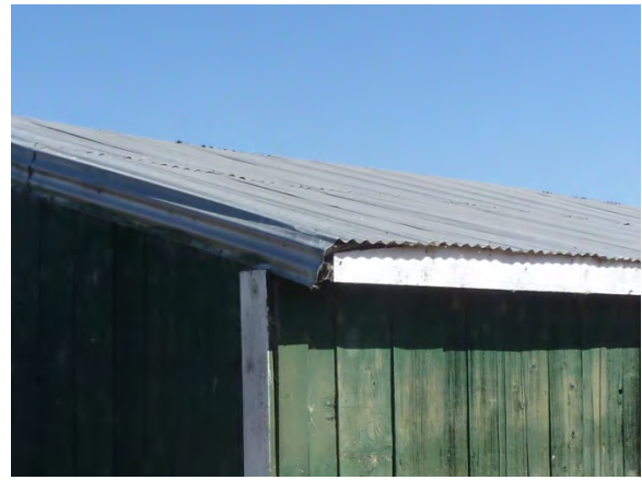
Image 71 - Metal Roofing, wrapped at gable end
