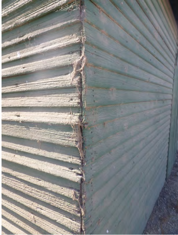
Image 109 - Siding at southeast corner of shed
