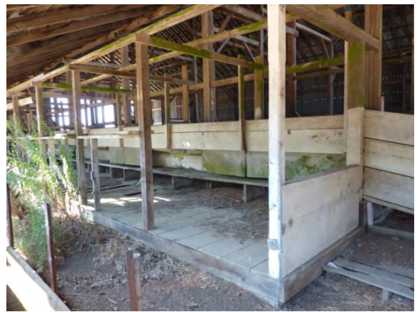
Image 64 - Stalls inside barn
