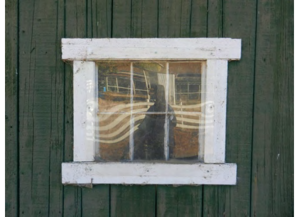
Image 119 - Typical window with plexiglas cover
