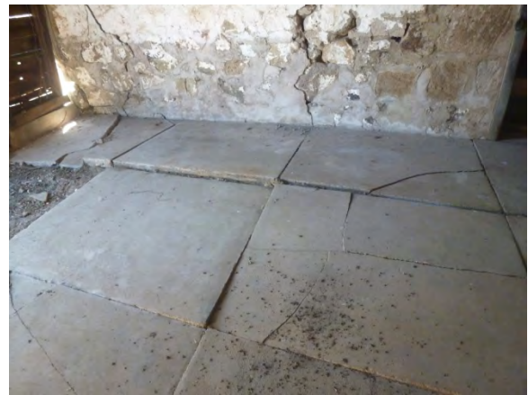
Image 76 - Floor slabs at mid-level of building
