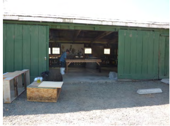
Image 125 - Large sliding doors to accommodate equipment.
