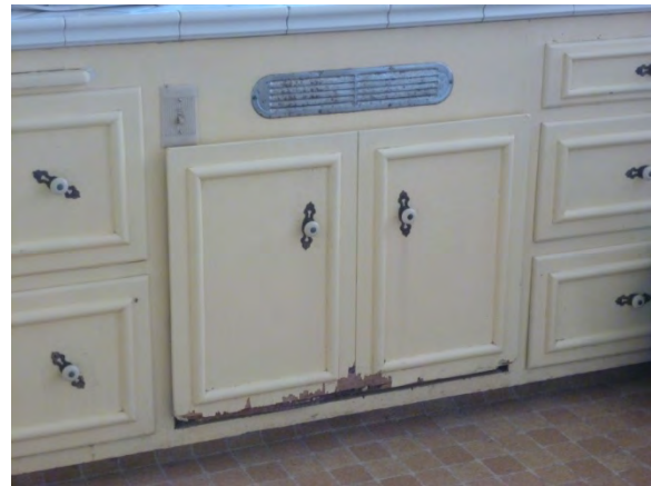
Image 43 - Cabinet at kitchen sink
