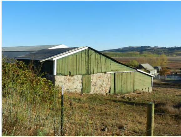
Image 65 – South wall of Creamery
