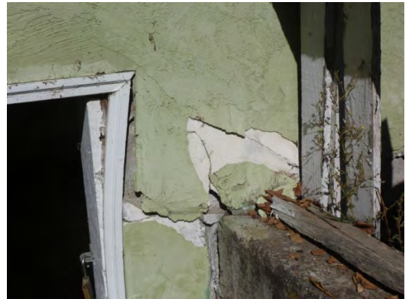
Image 18 - Stucco at basement stair and door
