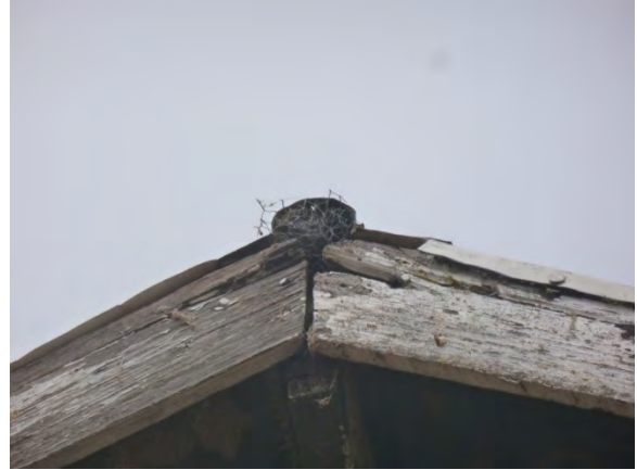
Image 87 - Roofing and trim at ridge, south end
