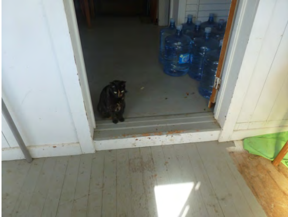
Image 8 - Step between enclosed porch and cottage
