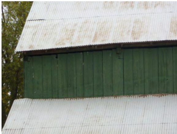
Image 49 - Typical condition of roof
