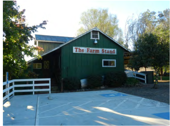
Image 79 – North end of Granary
