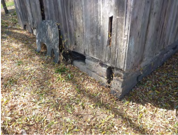
Image 99 - Building set on wood skids directly on ground
