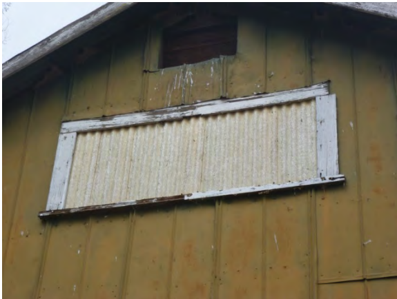
Image 90 - South Gable window with fiberglass infill.
