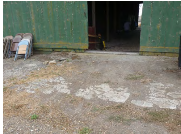
Image 54 – Stone and concrete paving at north entrance
