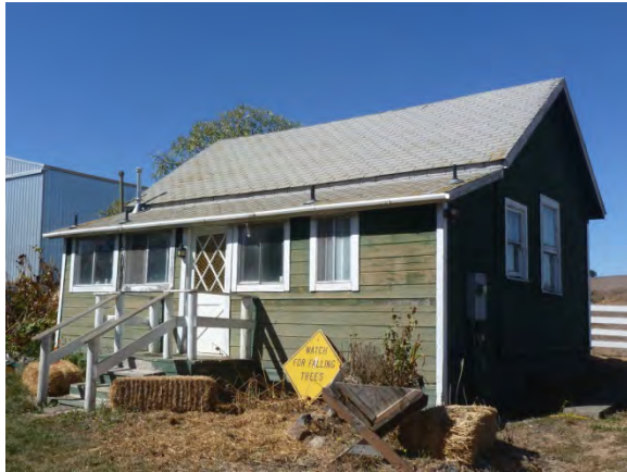
Image 1 - Entrance to Cottage, south side
