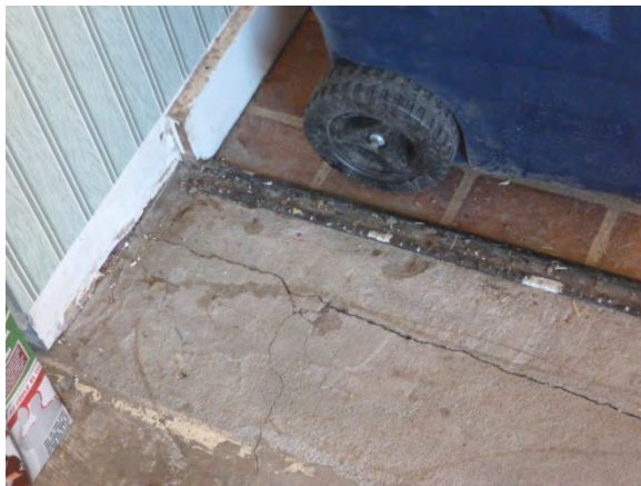
Image 41 - Floor at former garage
