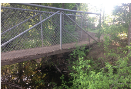
Existing pedestrian bridge, west
