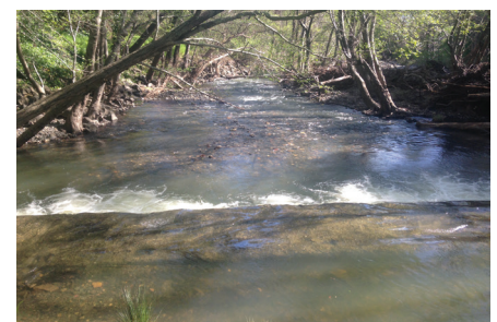
Sonoma Creek dam structure
