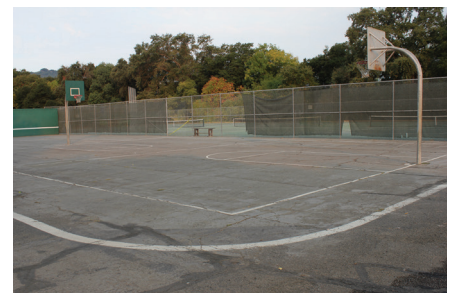
Existing basketball court
