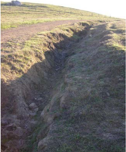
Photopoint 92. Erosion along road.
