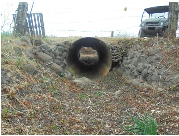
12. North Creek channel causeway culvert, looking southeast; notice top of culvert concaving from vehicle loads.
