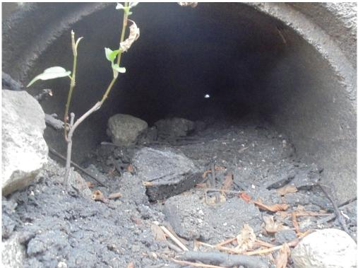
10. Looking southeast through Tolay Creek causeway culvert, ~70% full of sediment, but appears to be in good conditions.
